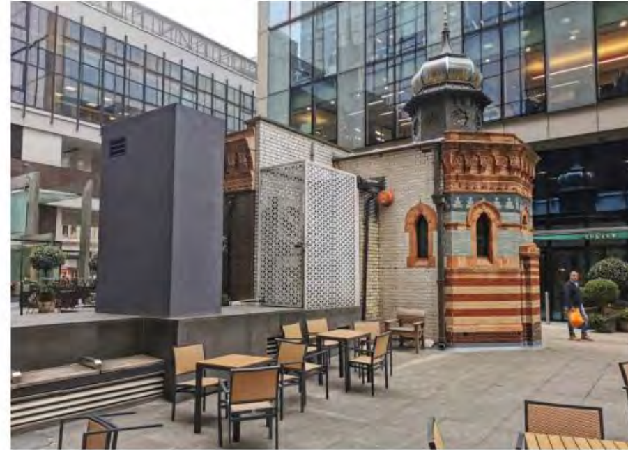
2 View from the King's Arms open space, showing the enclosed cage with kitchen ventilation.
