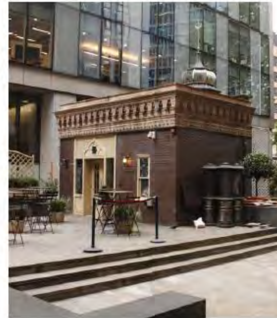
West elevation finished with engineering brick, extension made in the 20th century
