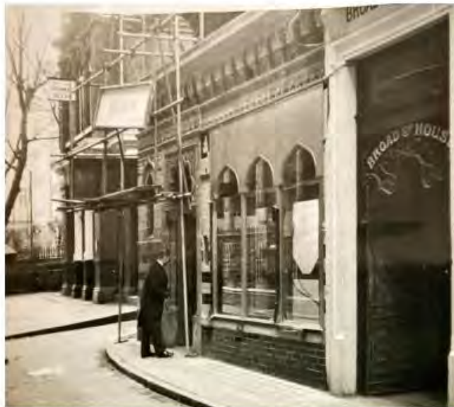
1 A 1968 photograph showing the kiosk to the Bath House and the neighbouring entrance to Broad Street House. The King's Arms is shown beyond. Scaffolding is present on the cupola to the Bath House indicating some repair works.
