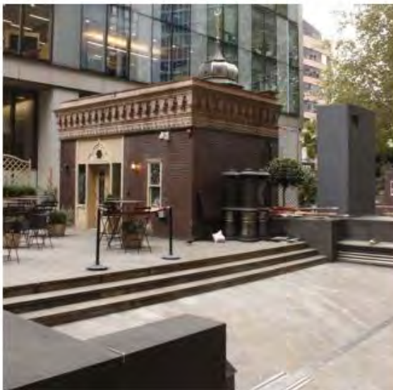
3 Existing public realm showing the 1970s extension to the Bath House.
