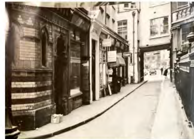
2 A view west showing the Bath House and adjoining shops, prior to their demolition.
