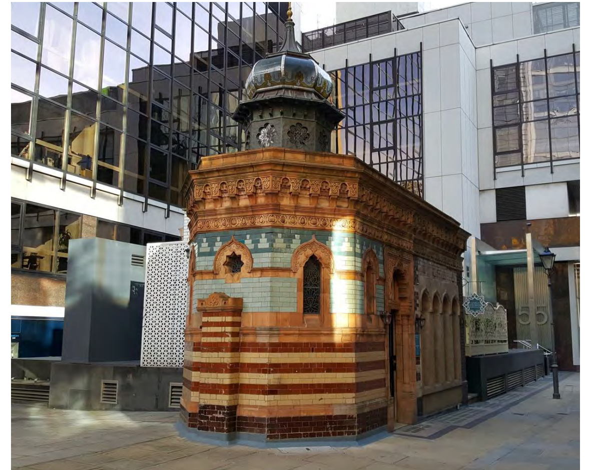
Existing poor quality modifications and surroundings
