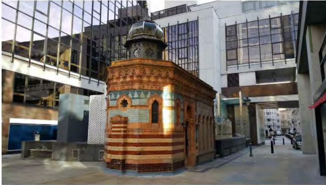
1 View west from public right of way
